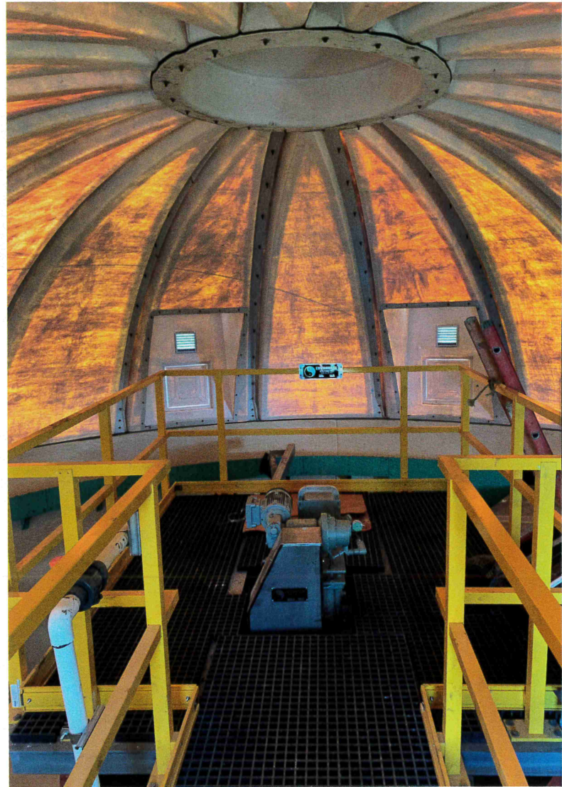
Completion of the mechanical equipment installation, catwalk, and access platform in Concentration Tank #4.
